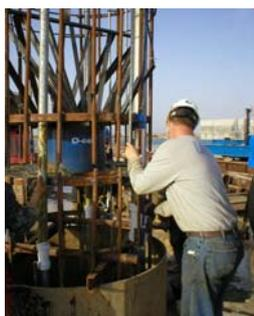
Installation of reinforcing cage with O-cell
